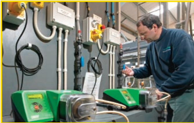
500 series pumps replaced high maintenance, high shear diaphragm pumps for coagulant dosing
