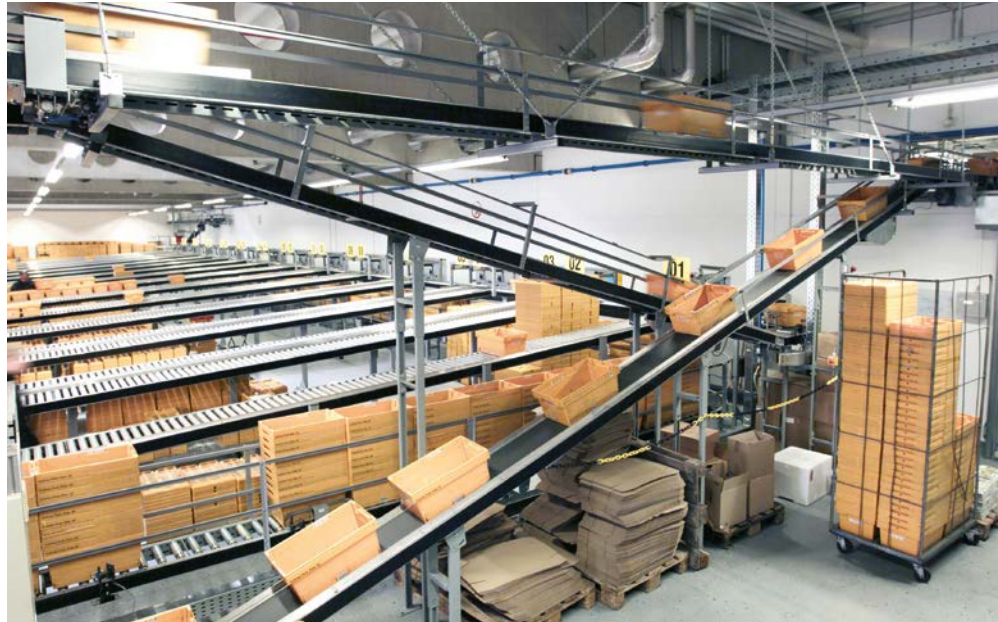
GOT1000 HMI's can help users see what is happening anywhere in their process.
