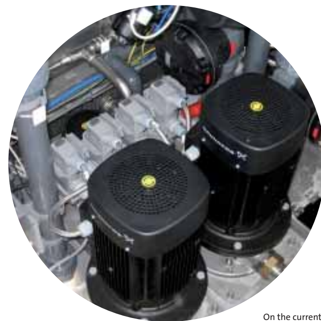
On the current ECM installations, Extrude Hone VMB is now changing all pumps to immersion pumps of the MTRI series, which also feature a stainless steel head.
