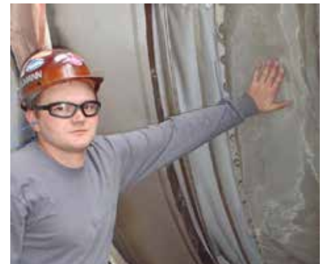
High temperature expansion joints may be designed to reduce surface temperature.
