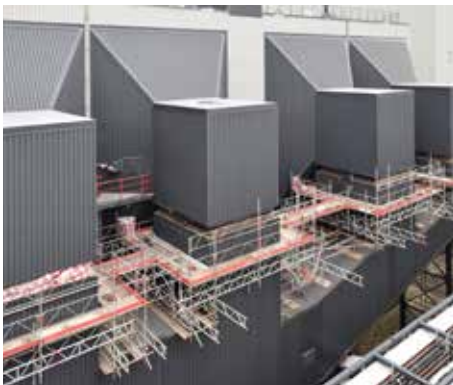
Fluaflex expansion joints being installed in boiler air intakes.
