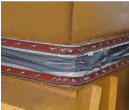
KE-Flex installed in an air duct.
