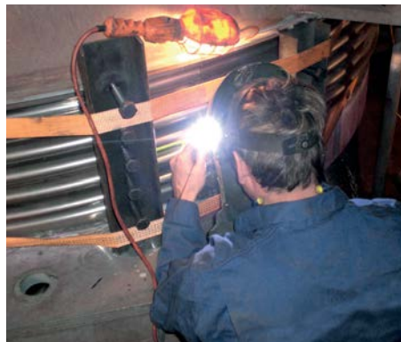
Installation of a clamshell metal expansion joint.
