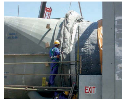
Installation of KE Fabric Expansion Joint.
