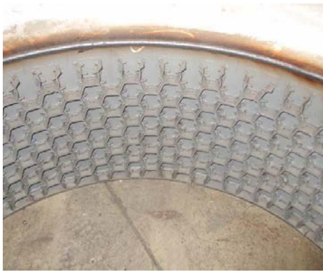
Hexmesh before castable material has been installed.
